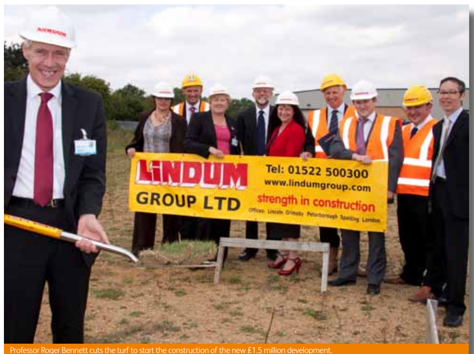
Professor Roger Bennett cuts the turf to start the construction of the new £1.5 million development.
